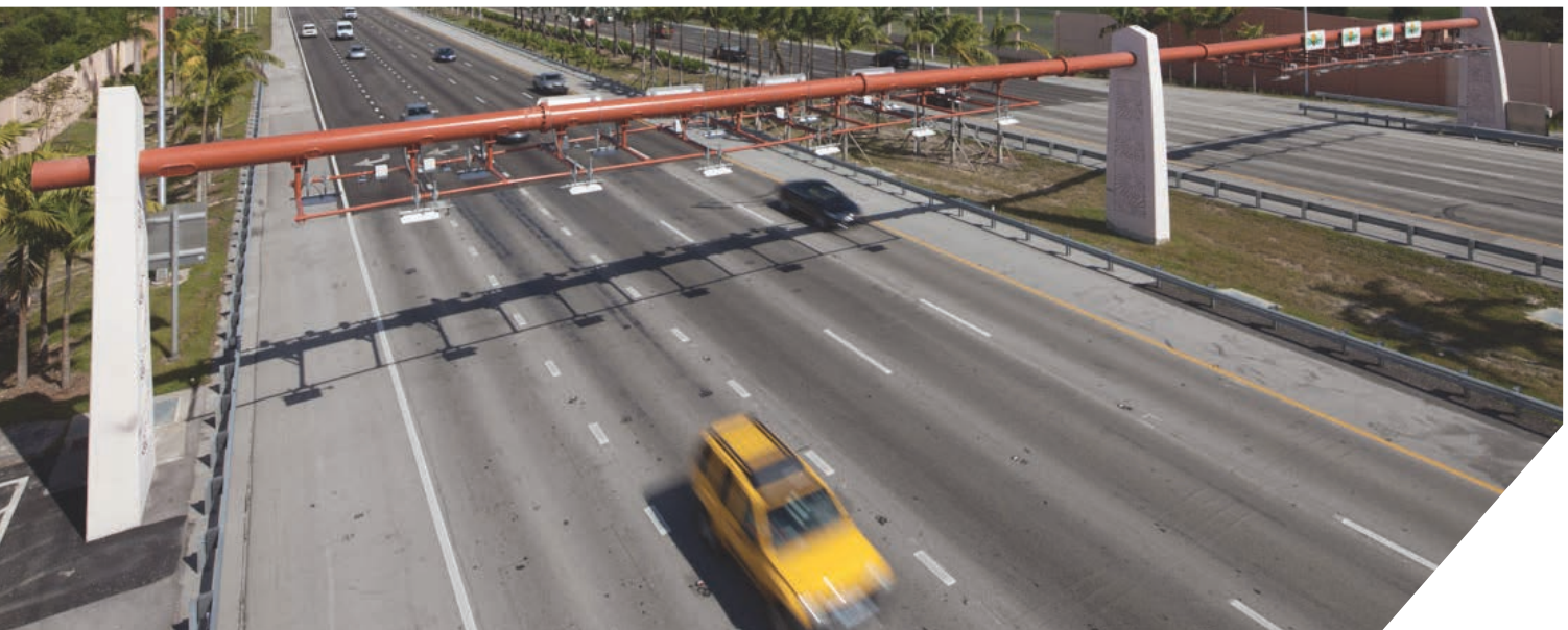
SR 874 Toll Gantry, ORT, AET
