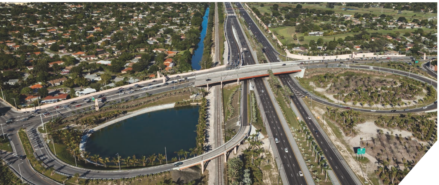
SR 874/Killian Parkway Interchange (Project 87404-000)
